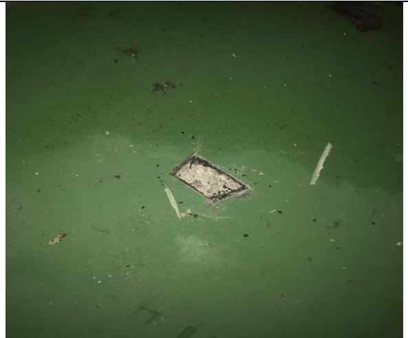
PIC.4 – Black foam under rubber floor - o concrete floor
