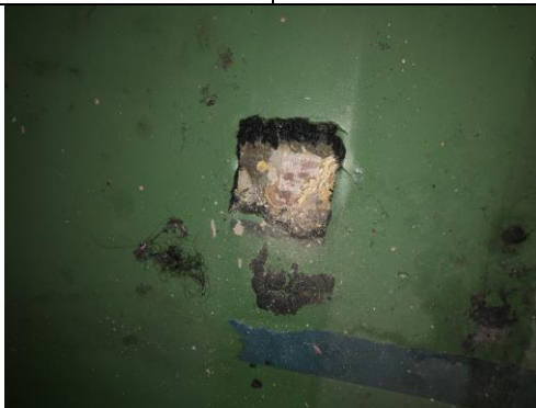
PIC.5 – Mastic under black foam on concrete floor
