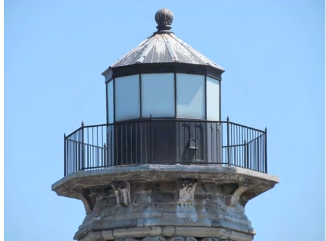
15. Lantern section set on deteriorated concrete platform.
