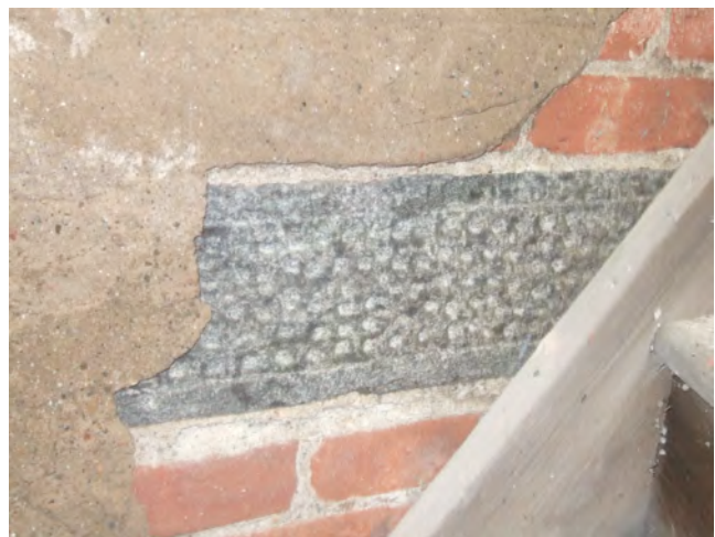
38. Detail view of loose stucco covering articulated trim stone.
