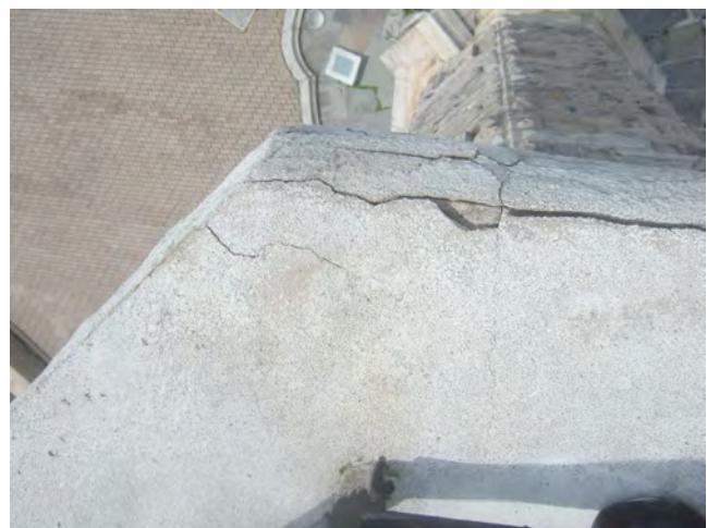
20. Loose section of concrete at south corner of platform.
