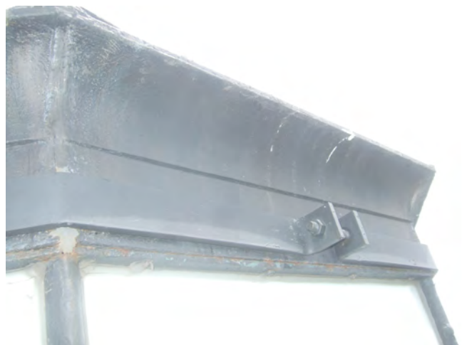
27. Strap at perimeter of lantern to prevent the spreading of the sections.
