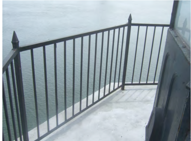
22. Iron railing mounted into concrete platform.
