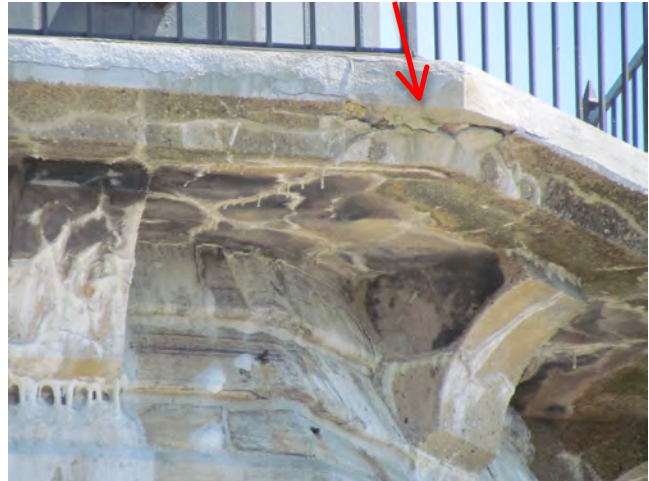
18. Cracks and efflorescence at concrete platform.
