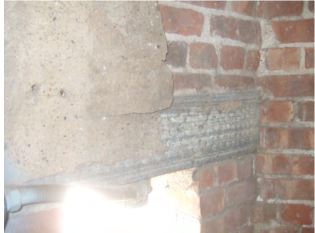
37. Eroded stucco covering original cut stone lintel.
