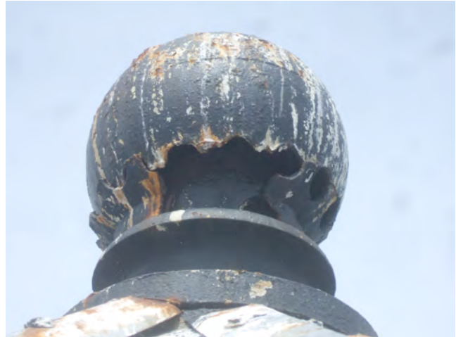
25. Broken ventilator orb at top of lantern.
