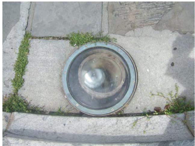
41. Deteriorated/nonfunctioning exterior light fixture.
