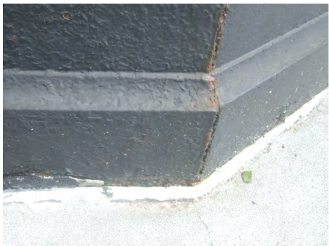
24. Typical open joint and rust at cast iron base sections.
