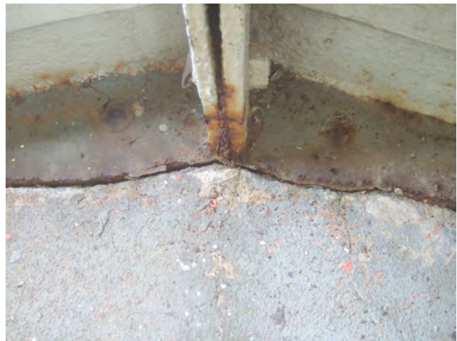
32. Rust and deteriorated cast iron at interior of base.
