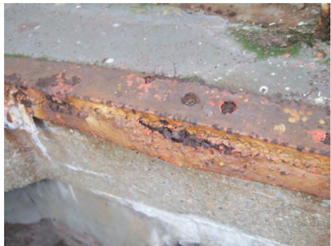
33. Deterioration metal flange at opening for access steps.
