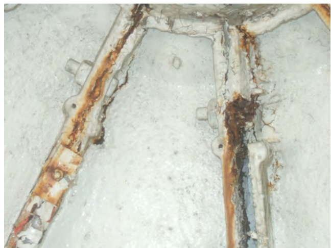
29. Detail of deterioration at center spoke of roof.
