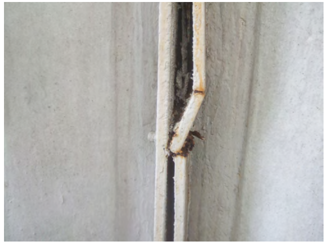
31. Cracked fastener and flange at typical cast iron base unit.
