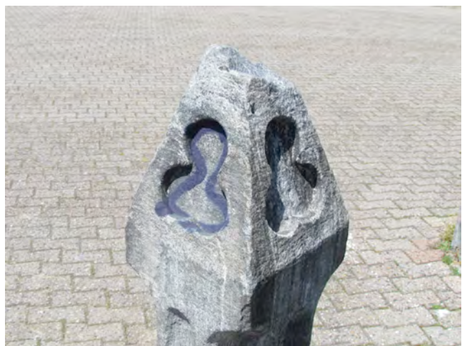
42. Stone bollard with broken tip and graffiti.
