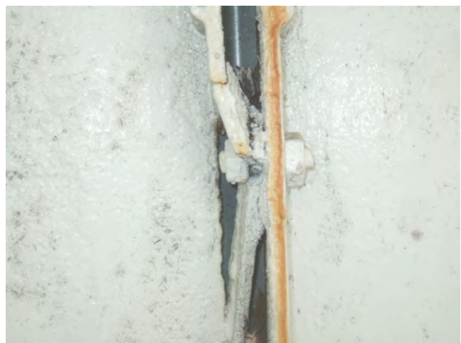
30. Cracked fastener and flange at roof section.
