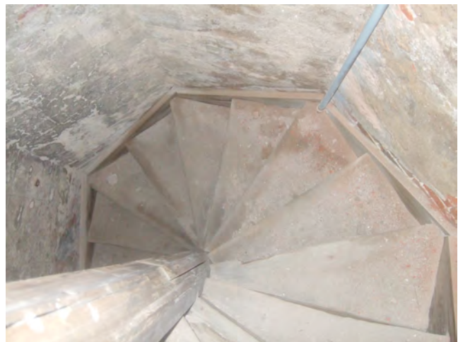
36. Spiral wooden stair with central wood post.
