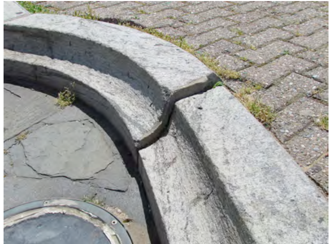
40. Displaced stone units at perimeter of stone paving.
