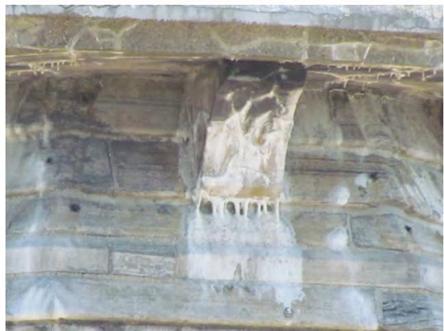
17. Deteriorated concrete bracket causing damage to stone units below.
