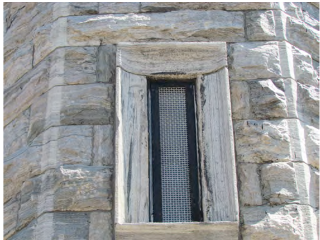
13. Lower level window with wire mesh screen.
