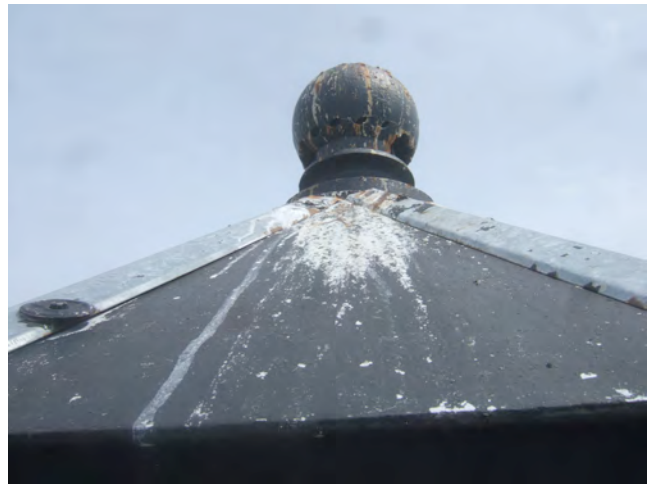
26. Stained lantern roof with deteriorated hip sections.
