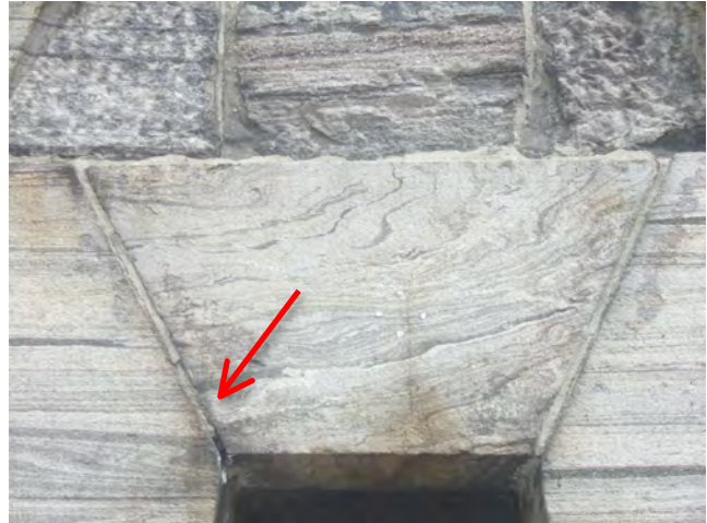
9. Eroded mortar joints at lintel stone.
