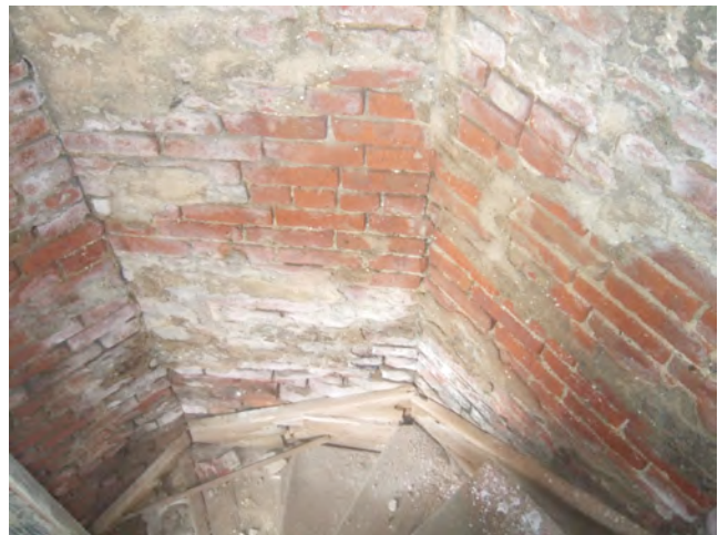
35. Deteriorated stucco and wooden stairs at interior.
