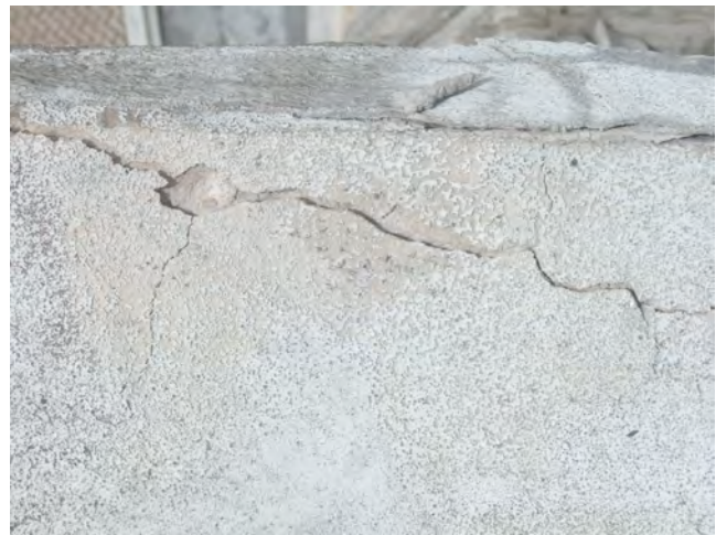
19. Open cracks and deterioration at waterproof coating at concrete platform.
