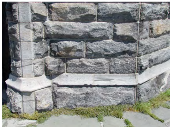
11. Base stone units with broken edges and open mortar joints.
