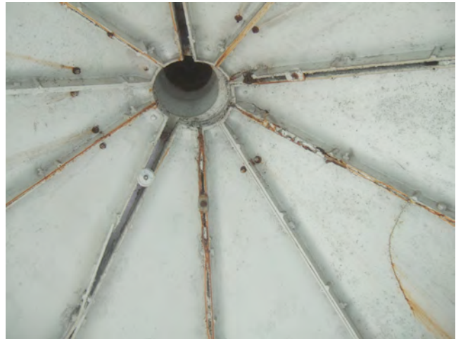
28. Deteriorated & cracked pie shaped roof sections separating from each other.
