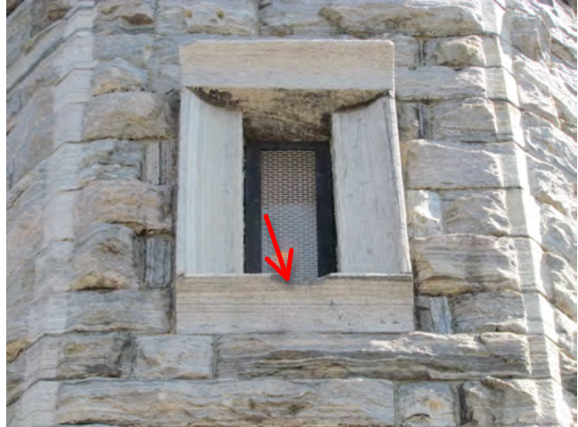
12. Upper level window with stone trim units. Note: broken edge of sill stone.
