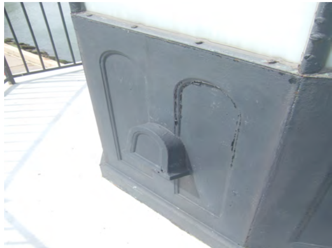
23. Lantern base section with ventilator.
